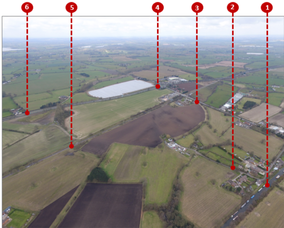
Figure 5: View looking north west across the part of the Site including the Canal (1), Croft Lane (2) the A5 (3), the Gailey Roundabout (4), the WCML (5) and the A449 (6) (March 2016)
